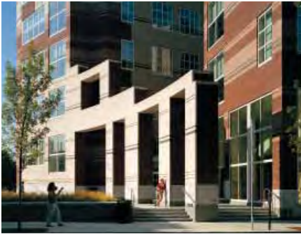
Front-side elevation and entrance arcade
